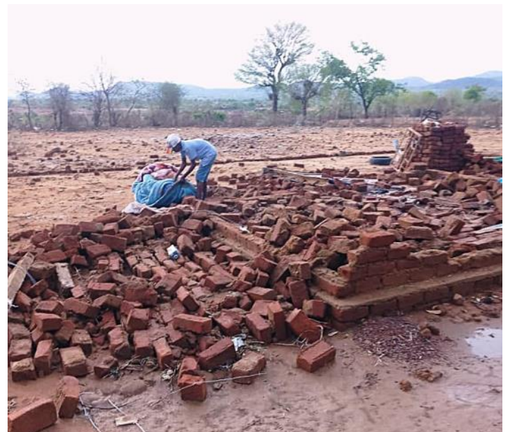
House destroyed by heavy rain in Mberengwa
